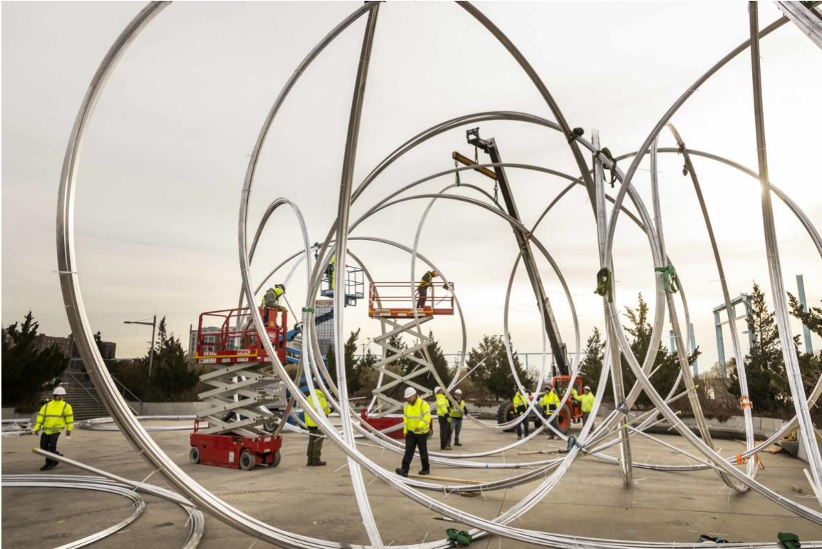
Workers installing New York Clearing. To adapt the piece from its gallery installation, where it hung with architectural support, to exist freely at Pier 3, Gormley relied upon a team of 25 to help anchor the work on the ground. Photo by Scott Rudd. © the ground. Photo by Scott Rudd. © the artist.
