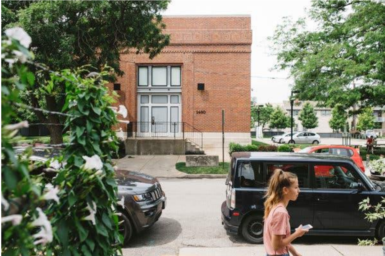
The Transformer Station in Cleveland, a museum that houses Mr. Bidwell's photography collection and is one of the staging sites for the triennial. Credit...Andrew Spear for The New York Times
