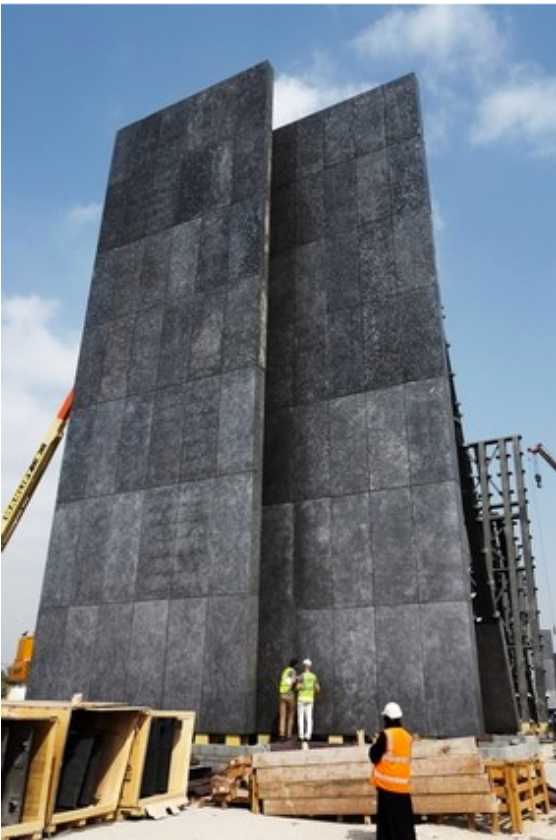
The memorial is made from hundreds of tonnes of steel. Its 31 panels and central spine are covered in 900 hand-painted, individually cast aluminium panels. Delores Johnson / The National
