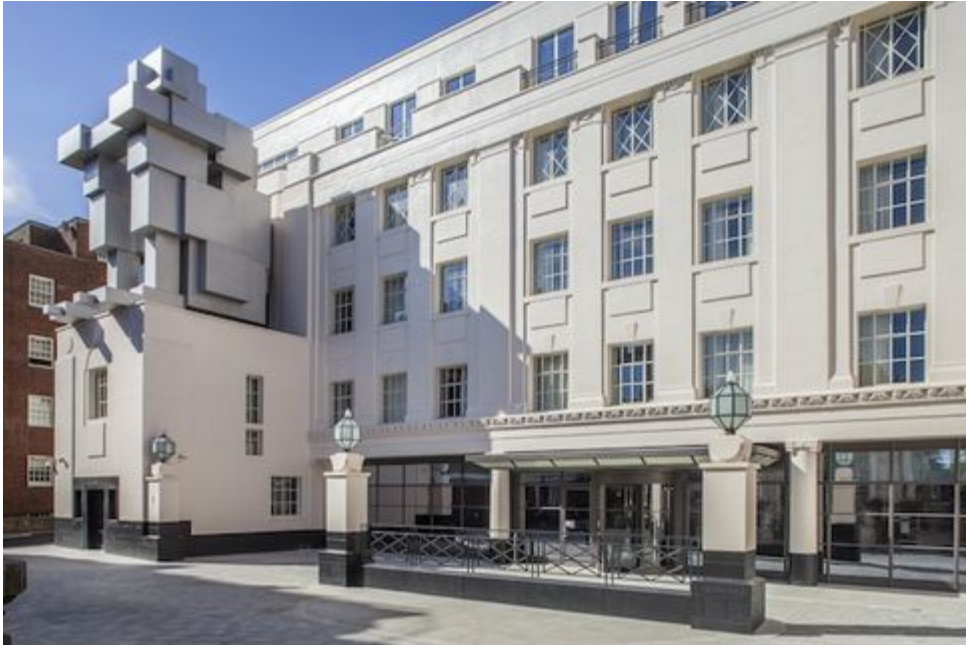
The exterior of the Beaumont Hotel.
